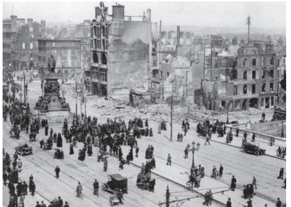
Devastation on Sackville Street, Dublin, where it crosses the River Liffey
